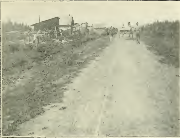
Tomstown, on the Blanche river, a new centre in northern Ontario. The Government road runs directly west into Evanturel township.
